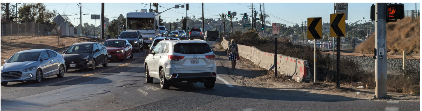
Missing pedestrian facility - signalized intersection has no connection with sidewalks
